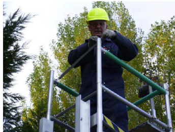
16. Once on the platform ensure the two (2) safety chains are hooked across the platform opening
