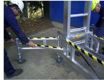
10. Clip on 2no. plan braces
