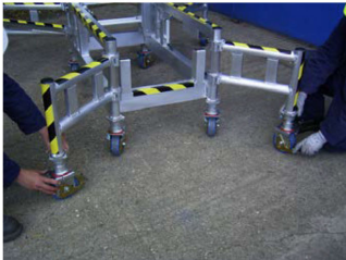
13. Adjust legs to level (use spirit-level) & lock castors
