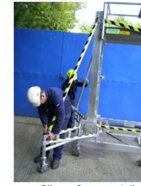
11. Clip on 2no. mast diagonal braces and tighten wing nuts on clamps
